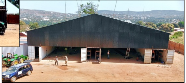
The new Joy in the Harvest Apprenticeship Training Center was donated and built by Don Reed of Open Door Enterprises and the team of eight from Kingwood (TX) Methodist Church .
