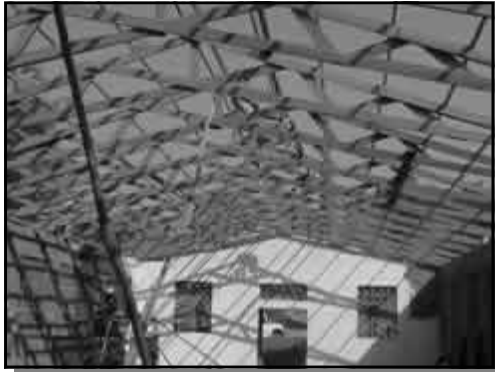
The new church at Gungu is ready for its metal roof.
